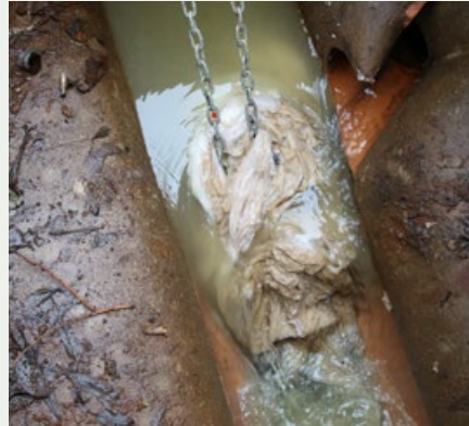
Our domestic misuse 'hedgehog' devices help to tackle blockages by capturing and removing unflushables, evidencing the scale of the problem.
