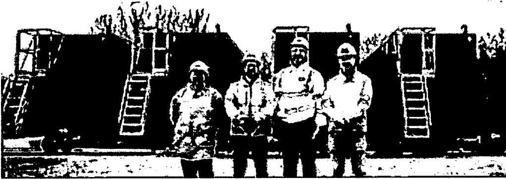
Submerged aerated filter units at Lower Moor Wastewater Treatment Works
