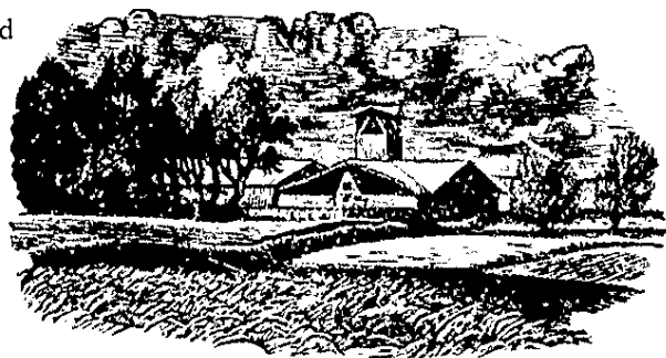
Ashford water treatment works, near Bridgwater
