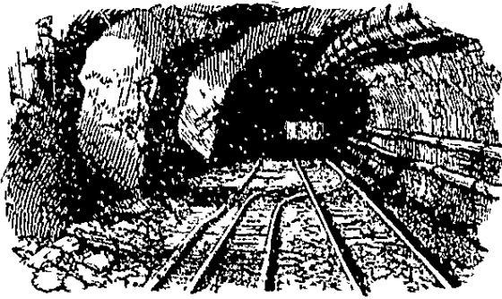
Construction of waste water tunnel, under Bristol
