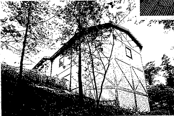
Dalarö, Stockholm, waste water treatment plant made to look like a summer house in an environmentally sensitive area. Interior above right.
