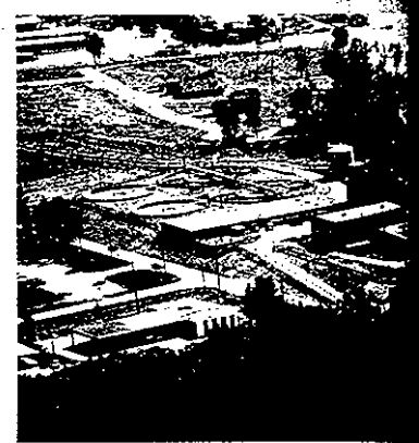
Water treatment plant, Evansville, Indiana, USA.
