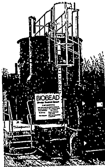
The Biobead process at Alconbury - In the forefront of technological development in sewage treatment.
