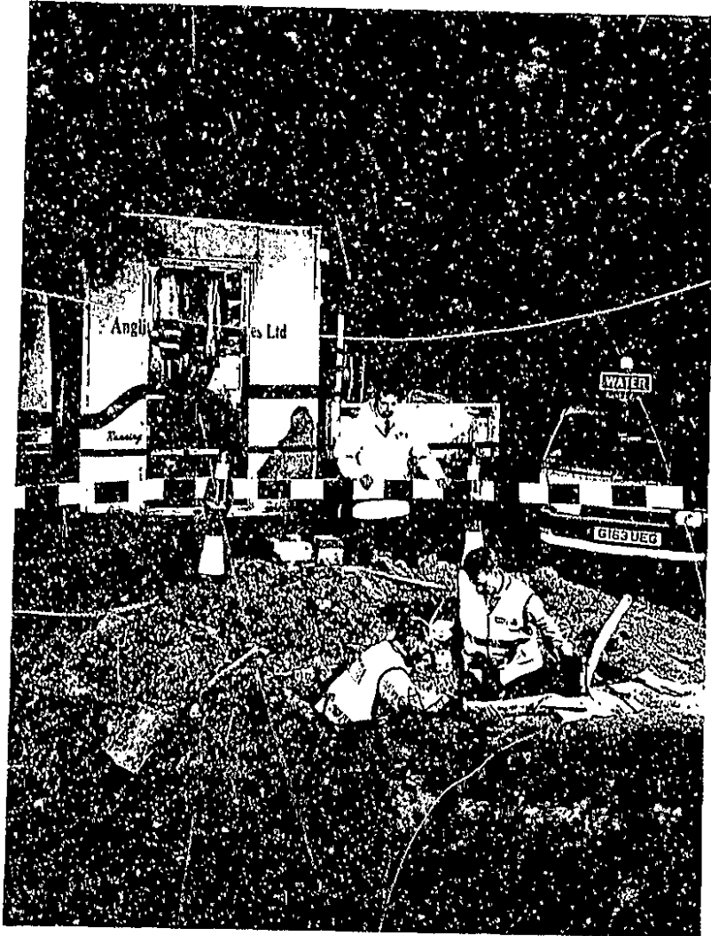
Our emergency service enables us to provide an effective response 24 hours a day - Shaun Arnold and Dave Lockey supervised by Inspector Nick Lilley carry out repair work.
