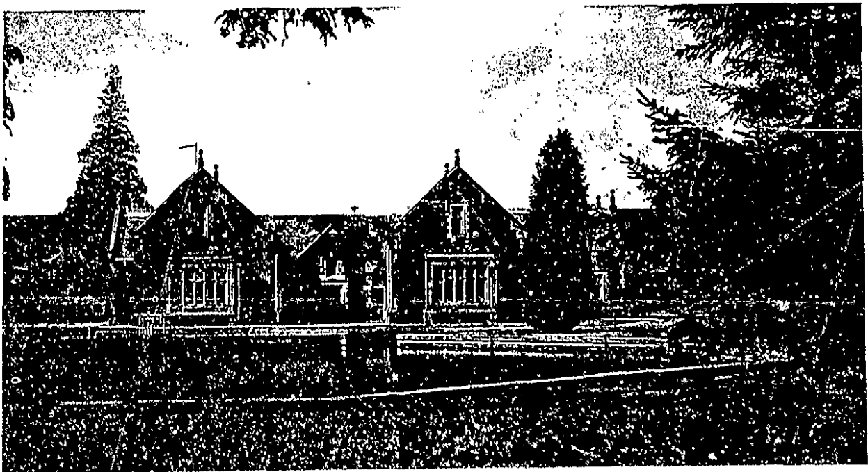
Ravenshorpe water treatment works (near Northampton) demonstrates how major operational activity can be carried out whilst maintaining the heritage of the building.
