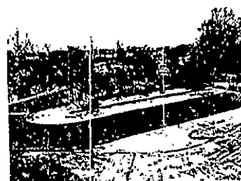
Activated Sludge Plant at Dunton (Beds.) - a modular design concept offering an economic form of construction for sewage treatment plants serving smaller rural locations
