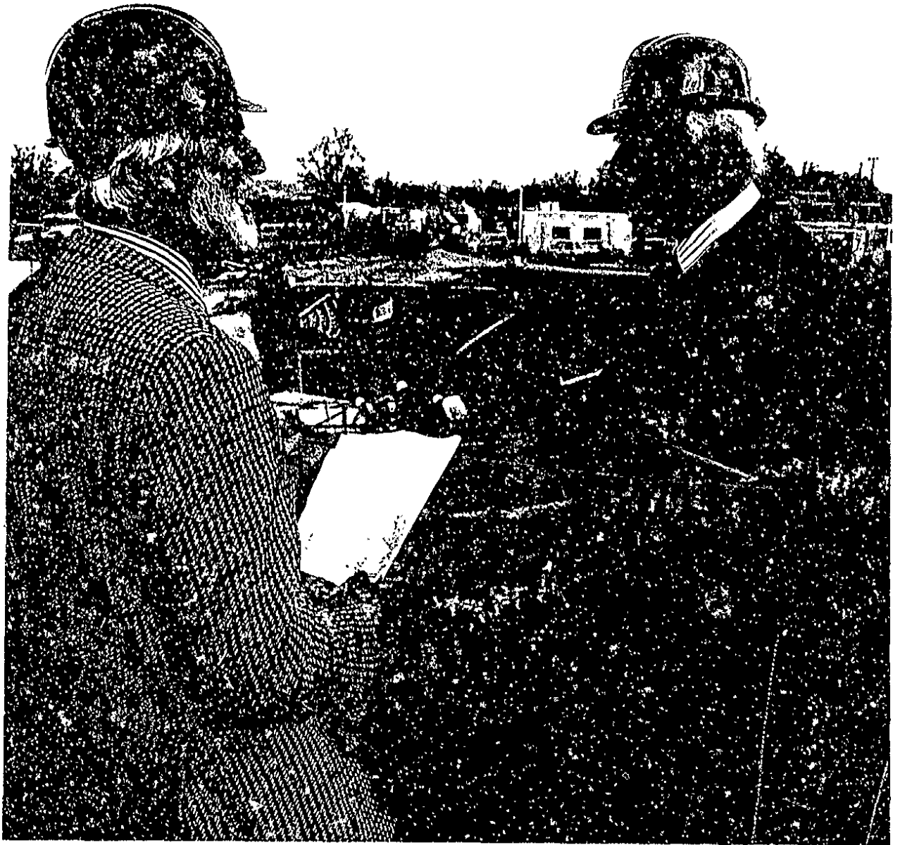
Chairman Bernard Henderson (right) discusses progress on the £1.2m extensions to Huntingdon sewage treatment works with resident engineer Michael Clack.
